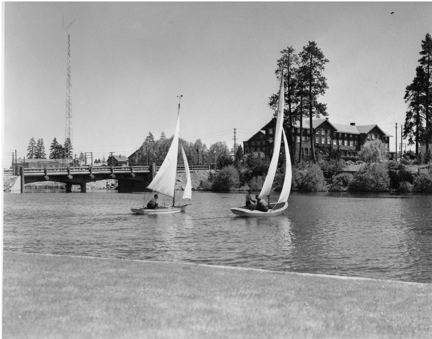
Newport Ave. Bridge, Mirror Pond, Pilot Butte Inn 1939
