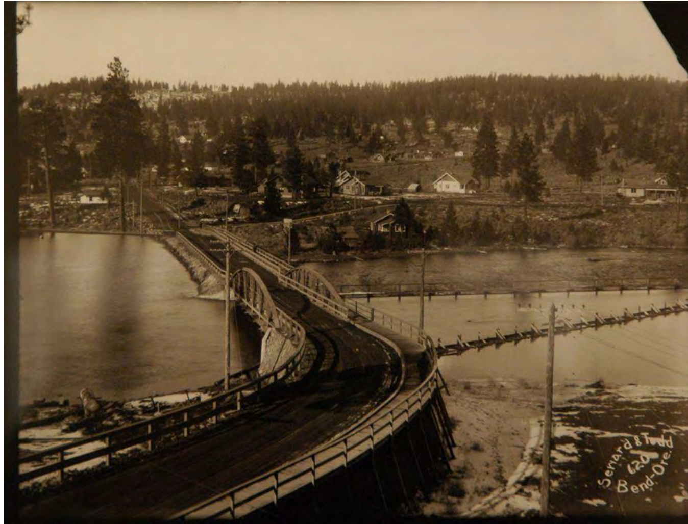
Newport Br.-Westside 1910s
