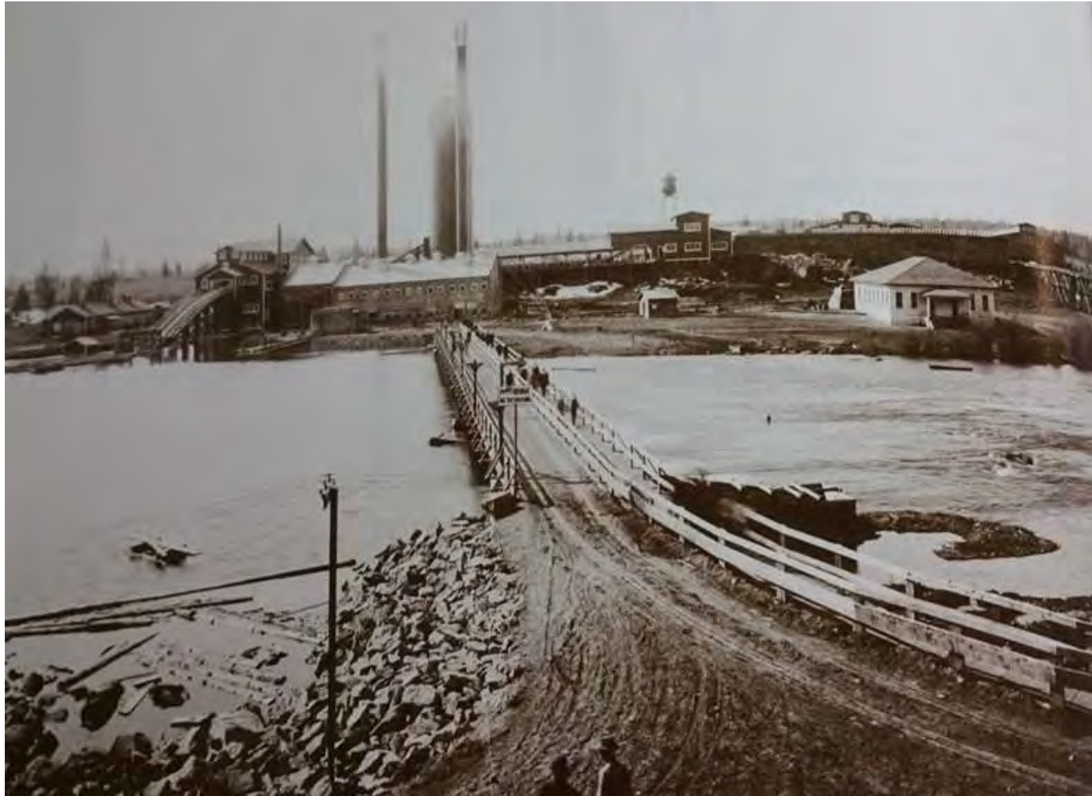
Shevlin-Hixon Bridge & foot commuters
