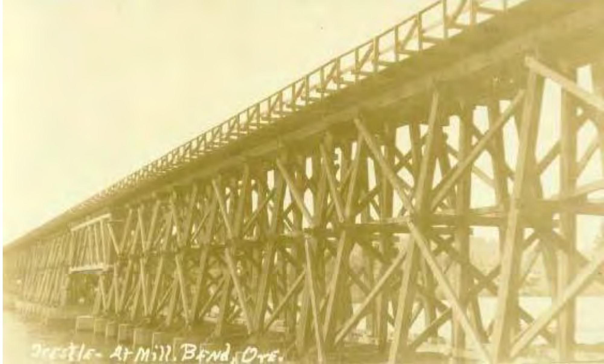
Trestle Shevlin-Hixon and Brooks-Scanlon Mills
