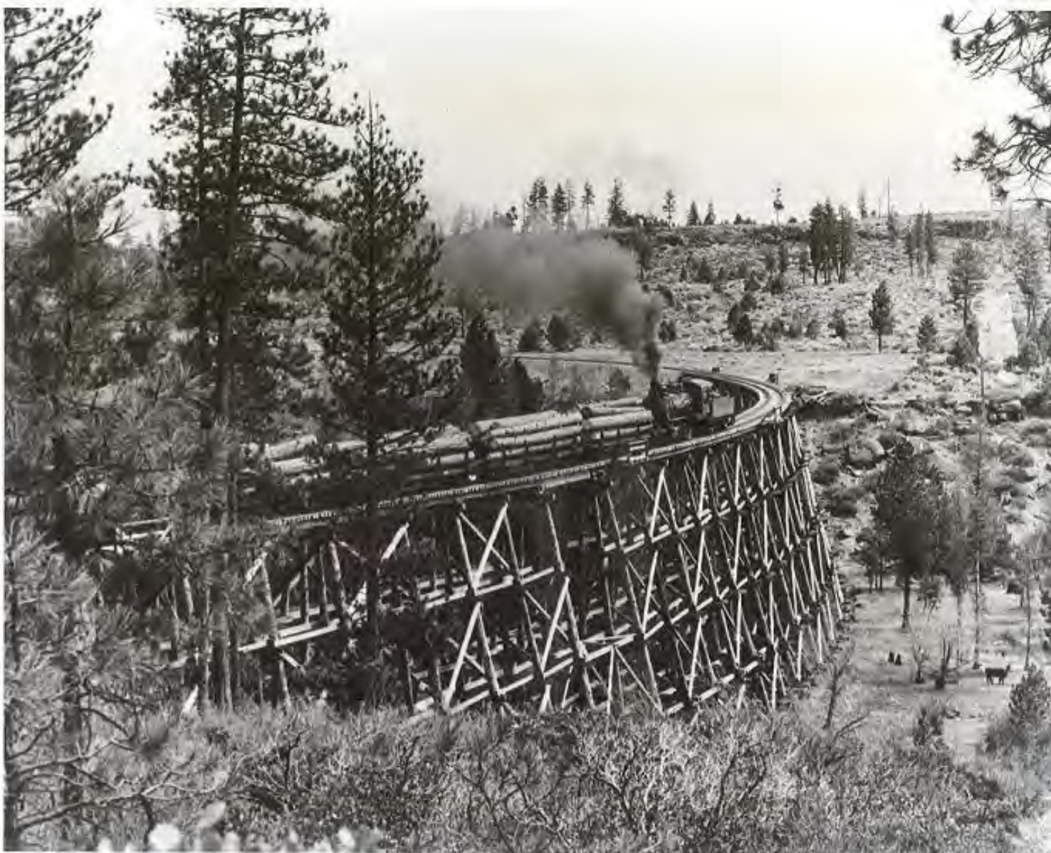
Shevlin Park Logging Rwy Trestle 1950s
